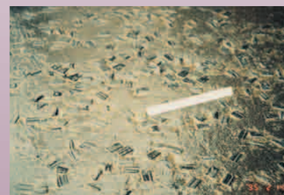
Finished pavement surface of "RUBBER ROLLED ASPHALT"
