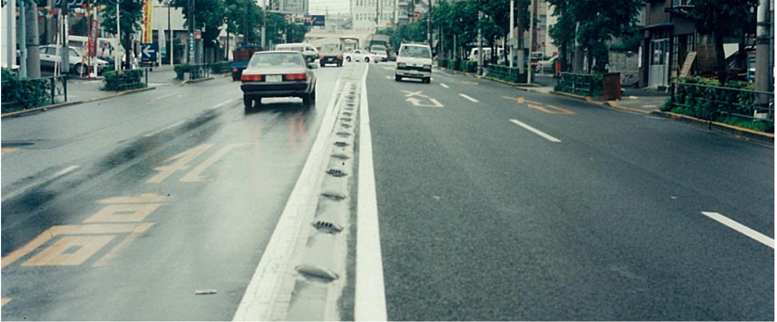
A city street on a rainy day (Left: conventional pavement Right: porous asphalt pavement)
