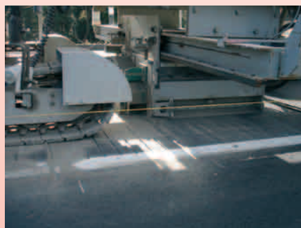
Grooving is formed perpendicularly to the traveling direction.
